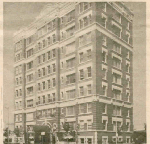
The Beaconsfield. 1700 Main Street. 1911. A. C. Pigg, architect. National Register nomination in preparation. (Paul Hester, Houston Architectural Survey. Courtesy of Houston Metropolitan Research Center)
