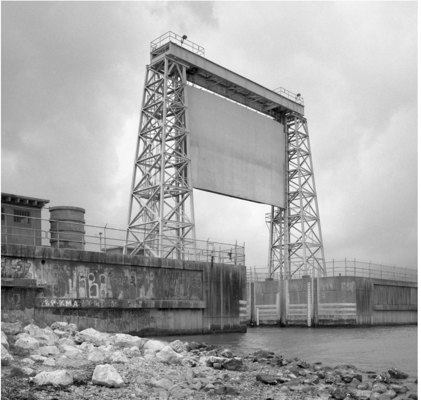
A guillotine-style floodgate marks the outlet between Moses Lake and the bay.
